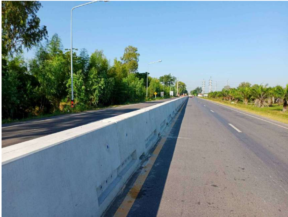
Single Slope Concrete Barrier
